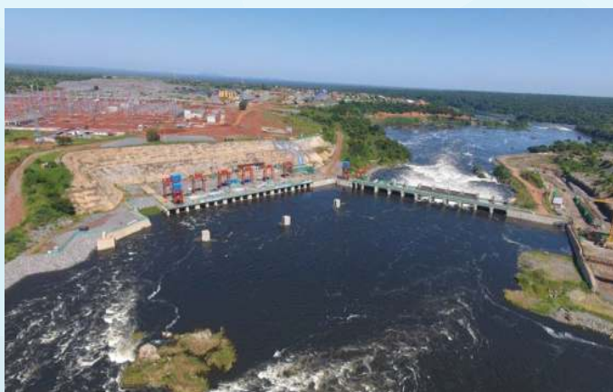
Karuma Hydro Power Dam 600MW
